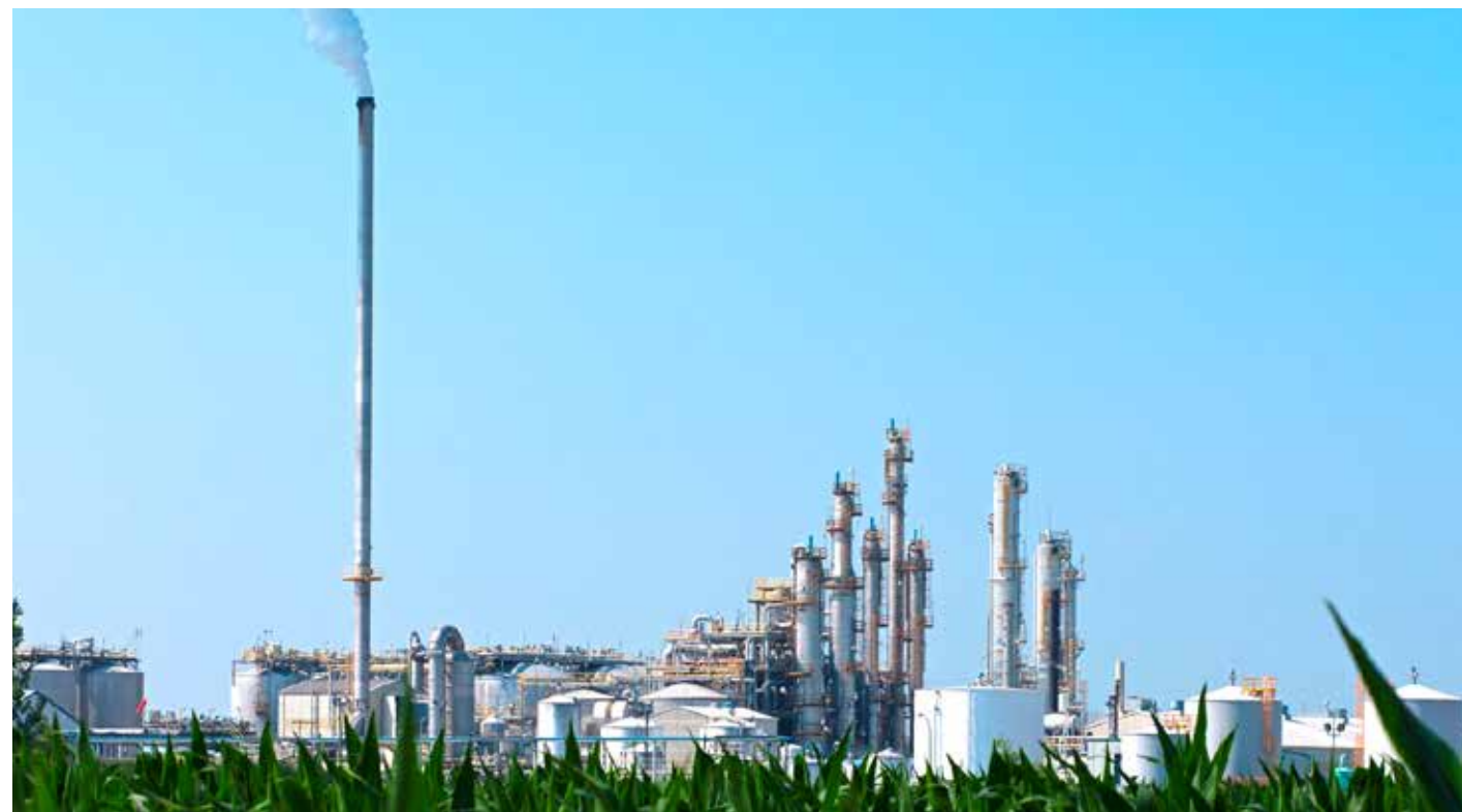
Pyroalliance makes equipment for petrochemical plants.
